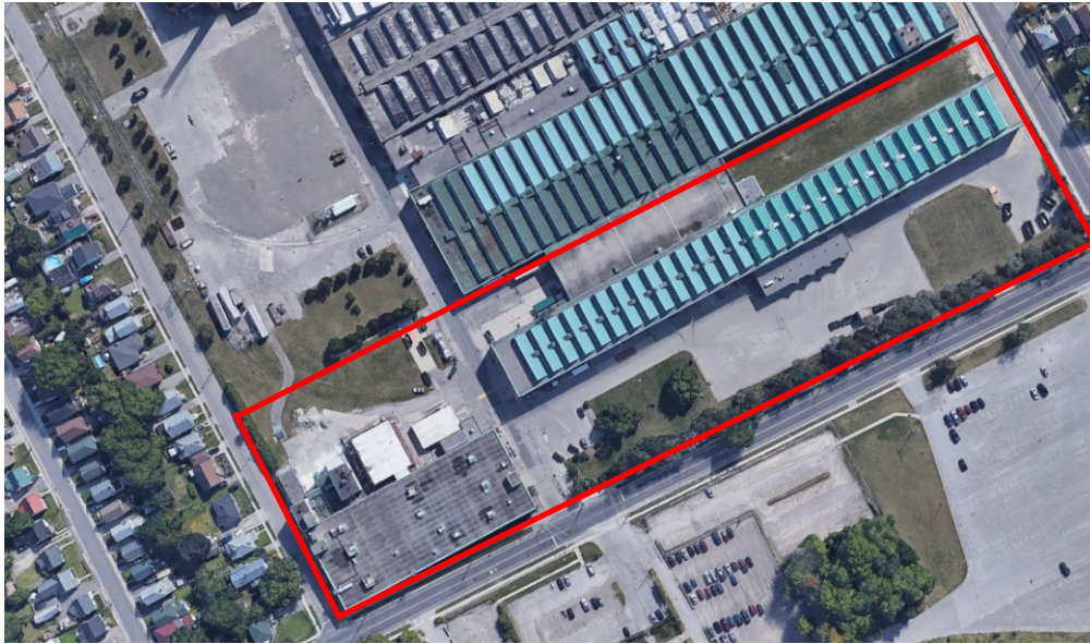
Figure 2-5: Aerial view of the BWXT NEC Peterborough facility (Source: Google Earth)
