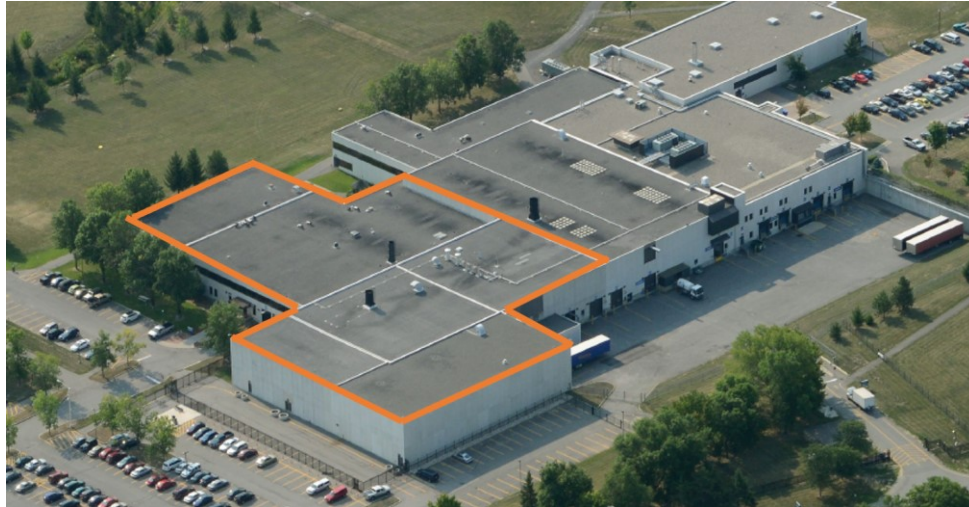
Figure 3-2: Aerial view of the Nordion facility (Source: Google Maps)
